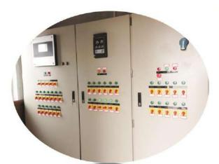
Electrical board of feeding system: The electrical installation and control board of feeding system consist of stop switches taking part on top and bottom parts, control cables and timer. Electrical board of manure removal system: These buttons are featuring sealed and self-protection system of engines. It is consisting of protective circuits and fuses of 2 pieces of engines with reducers of horizontal and vertical manure conveyors.
