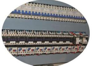
Electrical system and control board of automatic egg collection system. It is consisting of the protective circuits for automatic egg collection system, stop switches enabling the upwards and downwards movements of the lift stopped, control cables and control boards.
