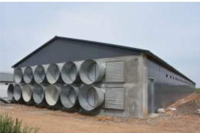
● The pullet chicken house are very strict to the temperature, therefore, we use the good box or cone fans and cooling pads in summer season and heaters (from Holland) to control temperature and give the pullet birds good feeling while rearing.
