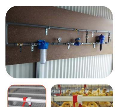
Easy drinking water management: is equipped with imported medicine pumps and filter, which can provide healthy water source for breeding.
