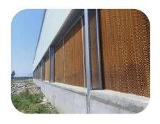
Equipped with cooling pads, the fresh air is cooled by the wet curtain and sent to the chicken house to provide moist air for the chickens.
