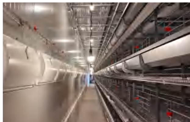
The even light distribution simulates the sunrise and sunset to improve egg production rate
